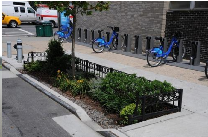
Curbside bioswale on city street, New York City, NY
