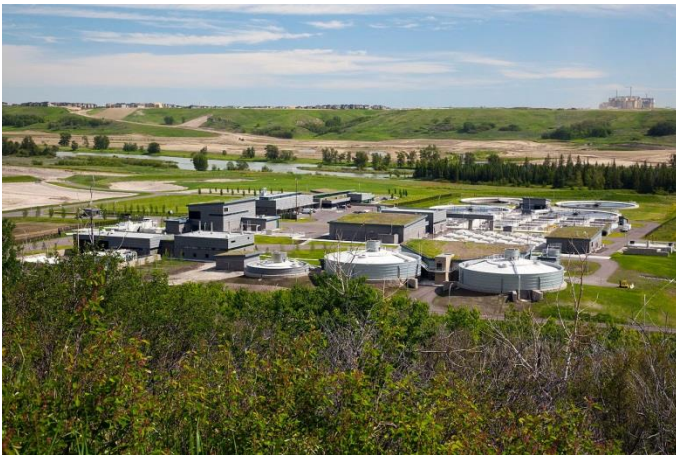
Pine Creek Wastewater Treatment Plant, City of Calgary
